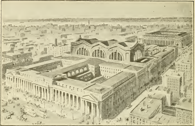
PENNSYLVANIA STATION. New Post Office in distance.
